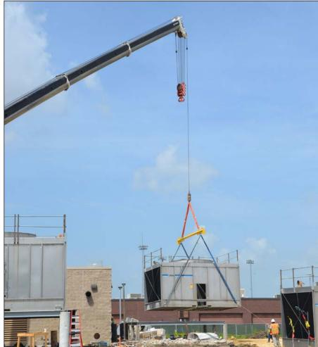
The construction crew at La Porte High School uses a crane to relocate a cooling tower on the site. The move was part of the process toward construction of the new Career and Technical Education Center at the campus.
