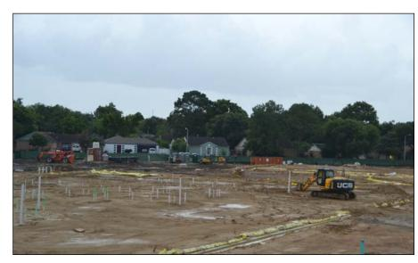
Plumbing has been installed and grade beams have been poured in preparation for the slab at the new Baker Sixth Grade Campus facility, which will be located south of the Instructional Technology Center on the current Baker campus.
