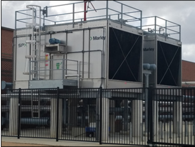
Elevated cooling towers at La Porte Junior High School. Photo courtesy of FEMA/Pamela Campbell
